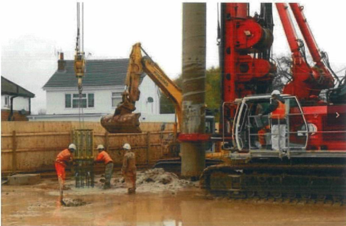
Fig 2.3 Photo of Piling Rig Operating Close to Houses – Similar to What is Proposed for Estuary Court
